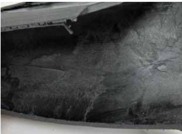
Figure 7: Photomicrograph of the cold flow fissures (white arrows) on the inside surface of the failed support.
