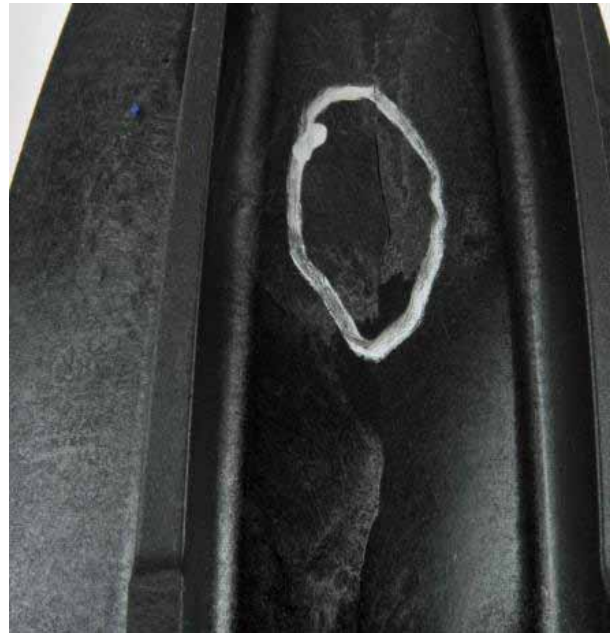
Figure 6: Close up view of the crack on the outside surface of the failed support.
