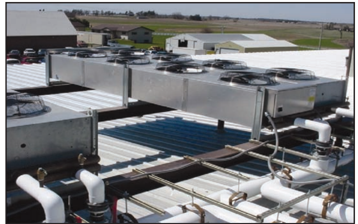
Winter-Kooler Unit on a roof.
