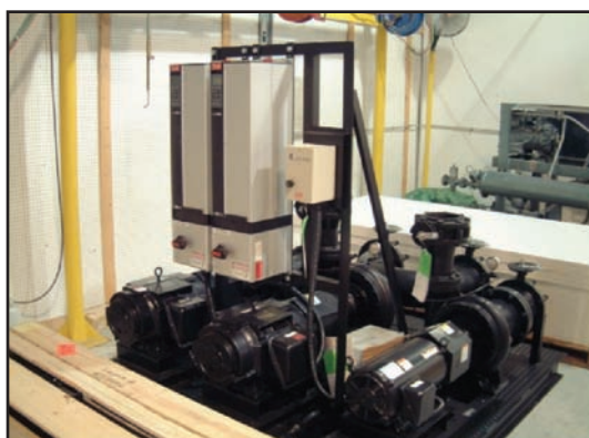
Variable Frequency Drive Pump Control. The smaller pump is the chiller pump.
