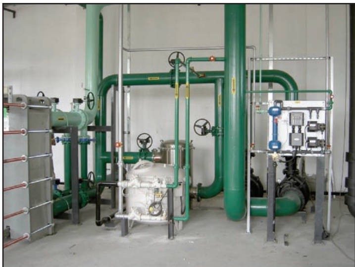
Closed Loop Tower System with Heat Exchanger (left) filters (center) tower water treatment unit (right).
