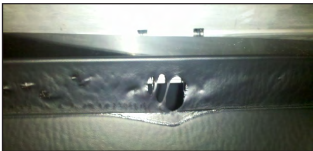
Figure 4. Tears in back of formed sheet.
